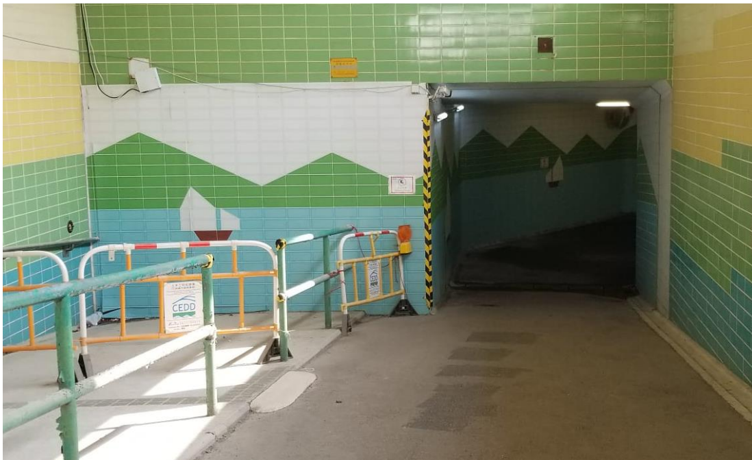
Photo 3 – Erection of site hoardings in unobtrusive colours
